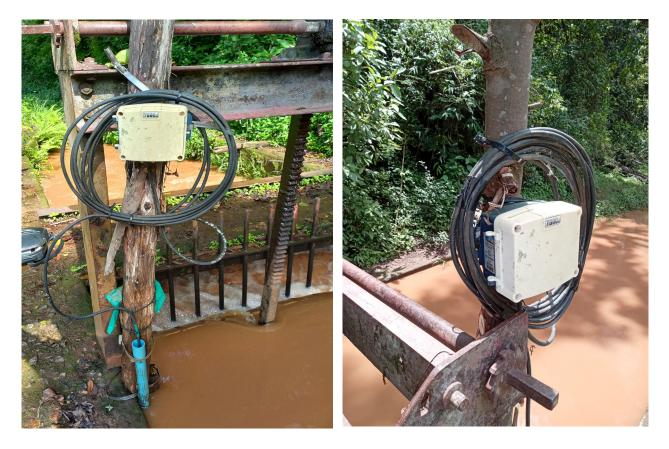
Figure 5 Water level logger at the Brewery Intake: on the left side before reinstallation, and right side after reinstallation.
